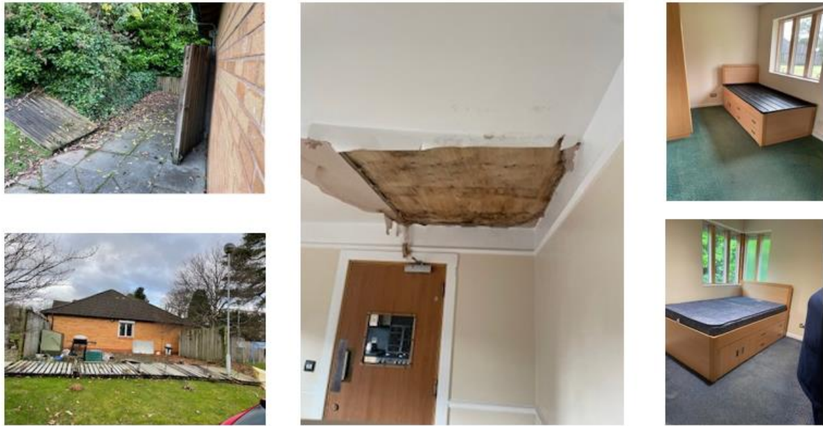
Figure 3. Photographs of the Existing Dan Y Deri Building
