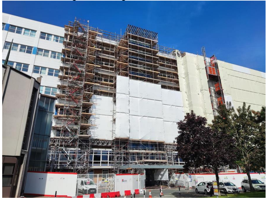
Phase 3 cladding scaffolding installation.
