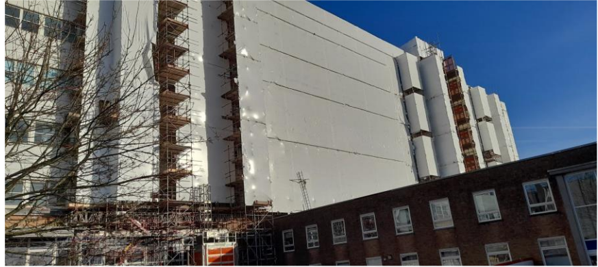
Phase 3 cladding scaffolding installation.
